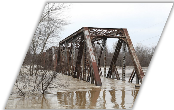
2015-2016 winter flood: Railroad bridge under water in Valley Park, Missouri
