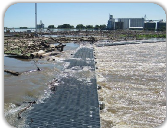
Flood water and debris at Lock and Dam 20 on the Mississippi River in Canton, Missouri, 2014
