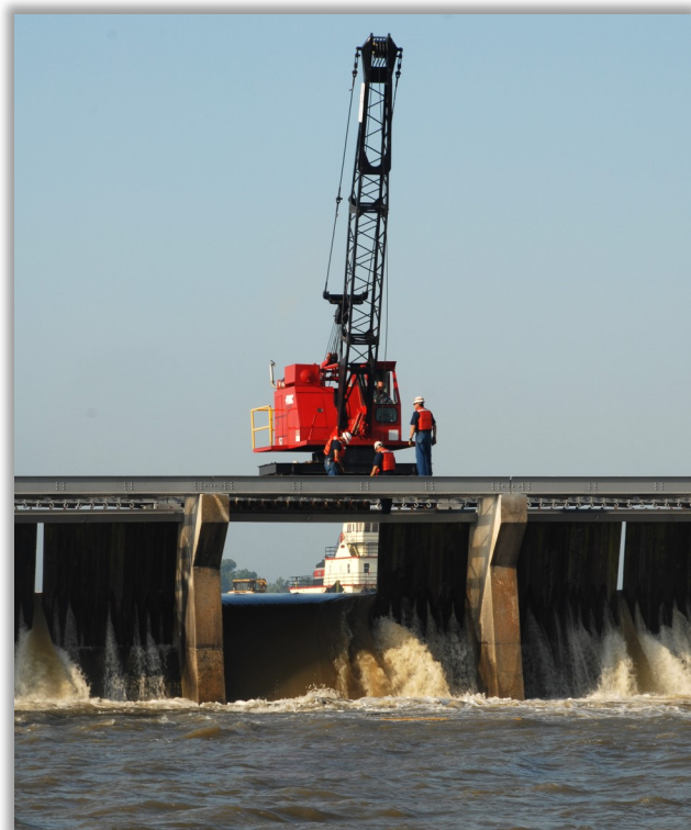
2011 flood: Raising needles at the Bonnet Carré Spillway
