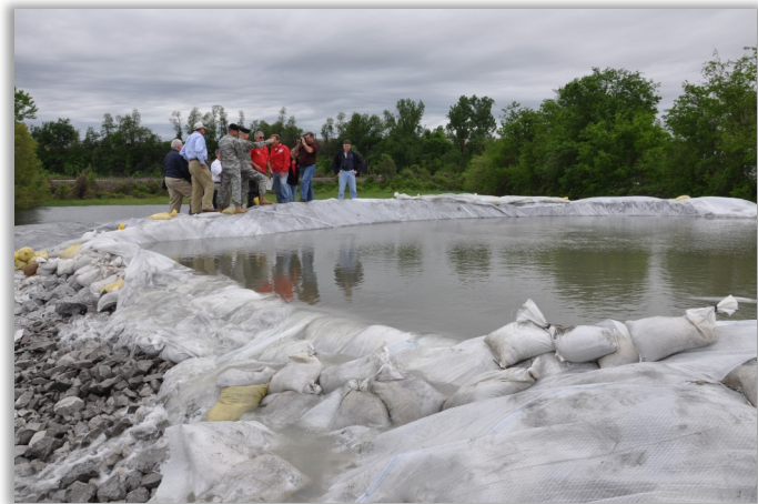
2011 flood: Sand boil at Cairo, Illinois
